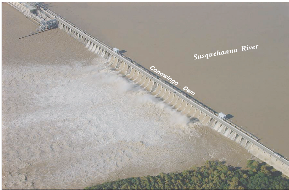
Figure 2. Release of water from the Conowingo dam on the Susquehanna River in Maryland on 21 September 2004 after Hurricane Ivan on 17–18 September 2004. The discharge is 384,000 cubic feet per second. This figure and the supporting data were adapted from Gellis et al. [2005]. The photo is courtesy of W. McPherson, USGS.
